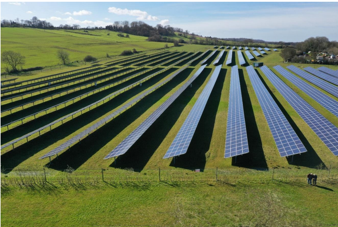
Image 1: Typical Example a of Solar PV Array
